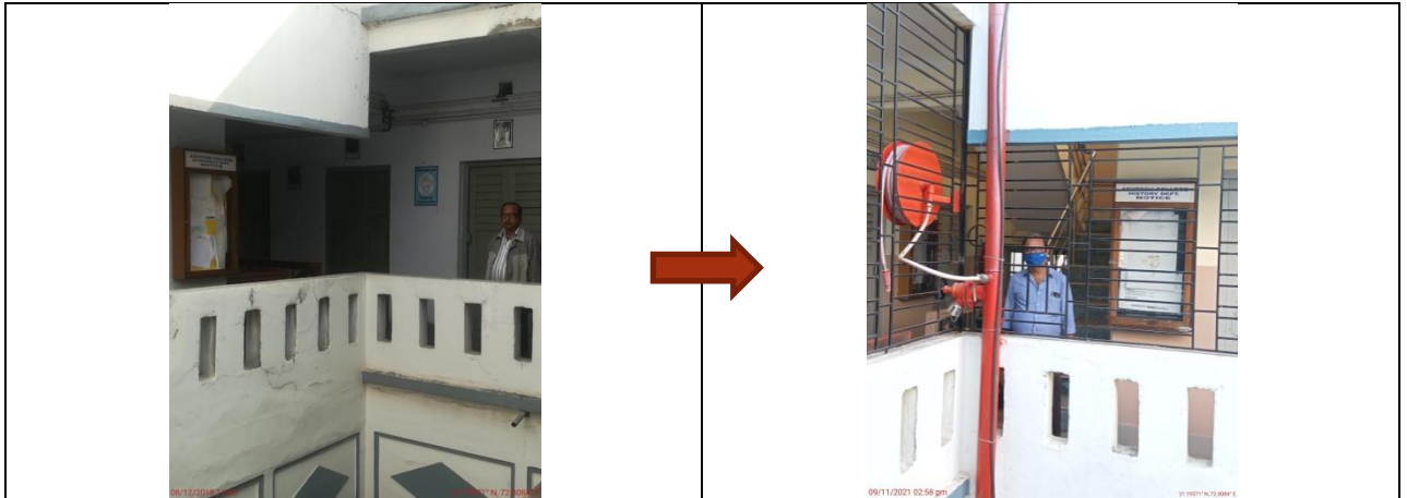
Installation of firefighting equipments and ducts. New grills.
