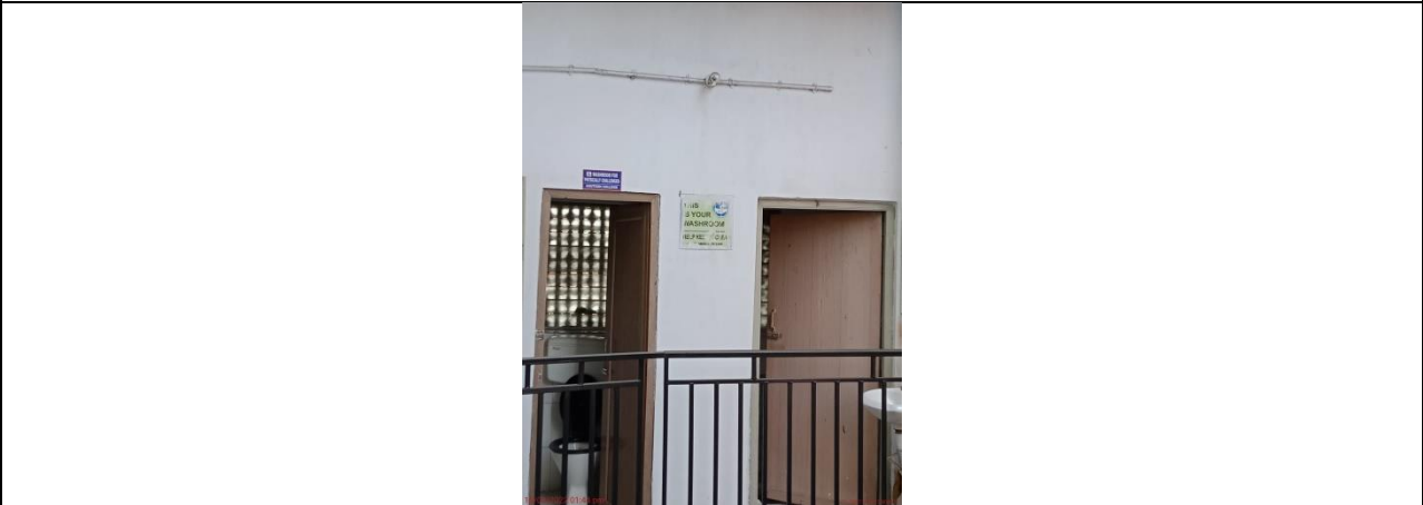
Renovastion of washrooms
