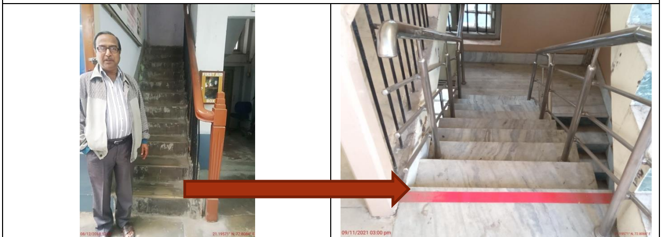
Staircase and railing
