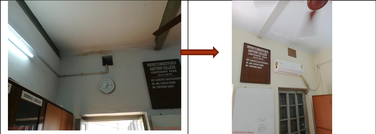
Renovation of Teachers' rooms and installation of AC
