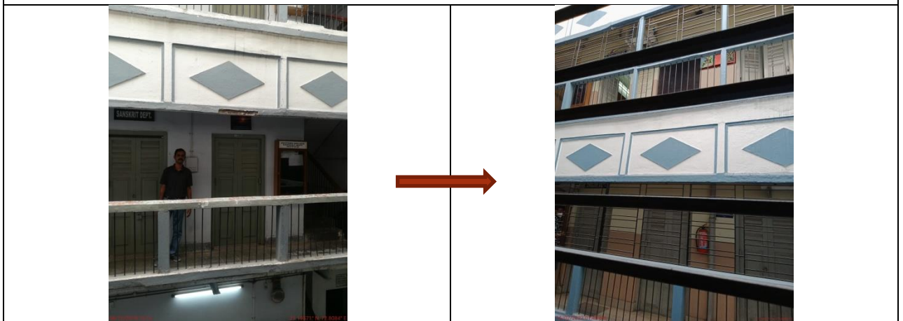
Renovation and installation of Grills
